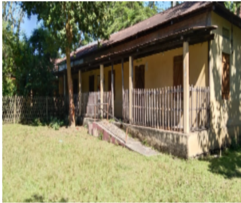
Polling Station Building Front View
