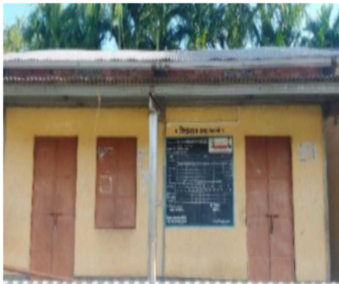
Polling Station Building Front View
