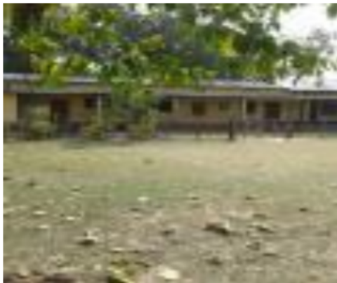
Polling Station Building Front View
