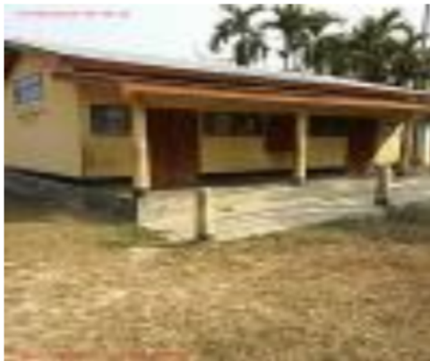
Polling Station Building Front View
