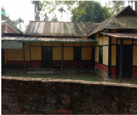
Polling Station Building Front View
