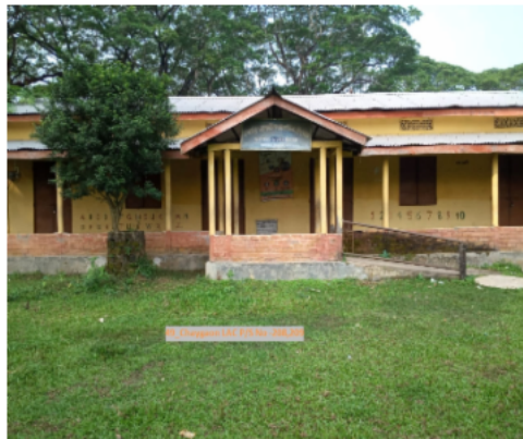
Polling Station Building Front View
