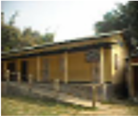
Polling Station Building Front View
