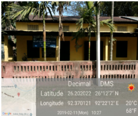
Polling Station Building Front View
