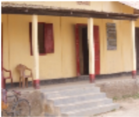
Polling Station Building Front View
