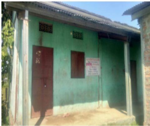
Polling Station Building Front View
