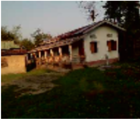
Polling Station Building Front View
