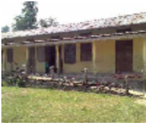
Polling Station Building Front View
