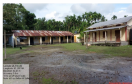
POLLING STATION BUILDING FRONT VIEW P.S. NO.-115
