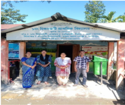
Polling Station Building Front View
