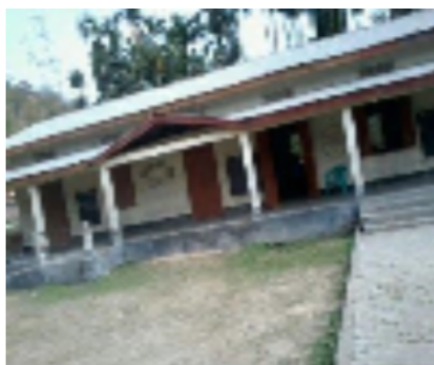
Polling Station Building Front View
