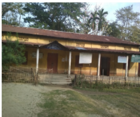
Polling Station Building Front View
