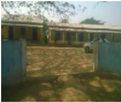
Polling Station Building Front View
