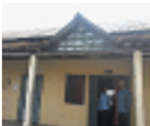
Polling Station Building Front View
