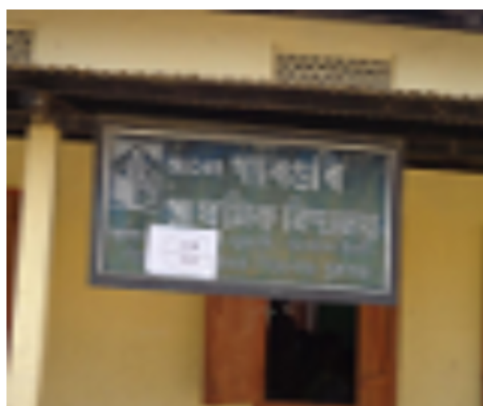
Polling Station Building Front View
