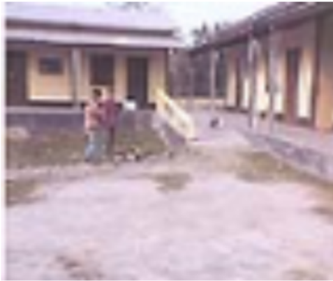
Polling Station Building Front View
