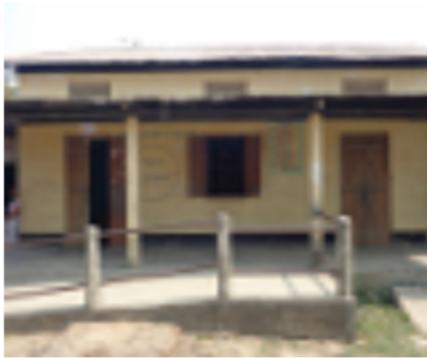
Polling Station Building Front View
