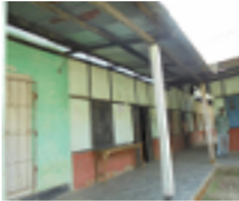
Polling Station Building Front View
