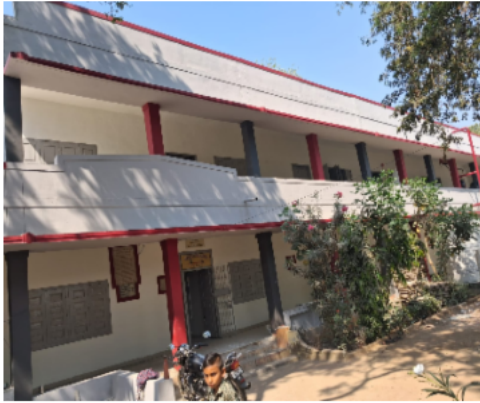
Polling Station Building Front View
