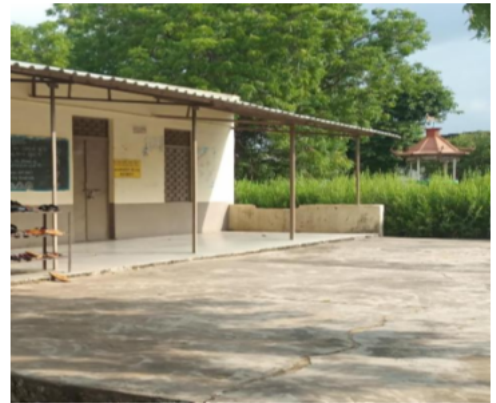
Polling Station Front View
