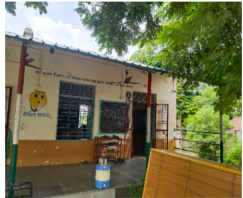
Polling Station Front View
