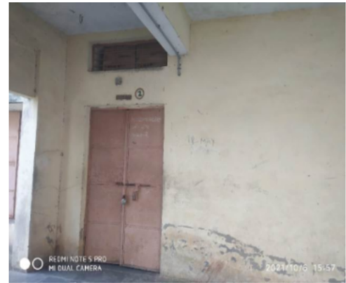
Polling Station Front View
