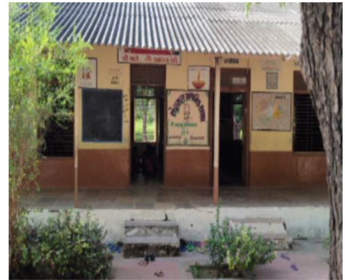
Polling Station Front View
