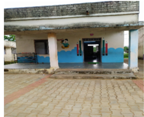
Polling Station Front View
