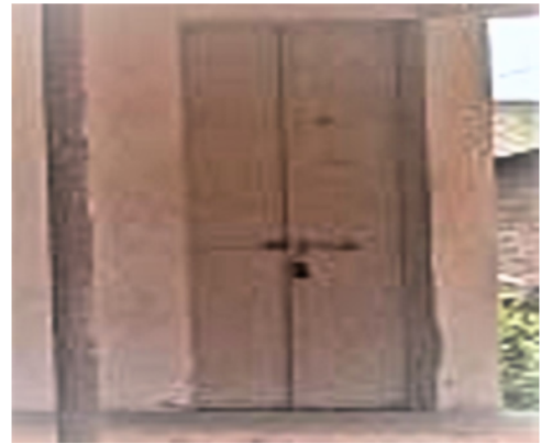
Polling Station Front View
