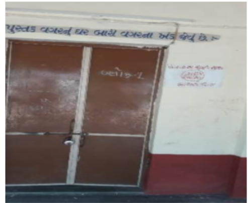
Polling Station Front View
