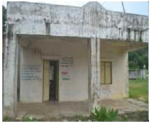
Polling Station Front View
