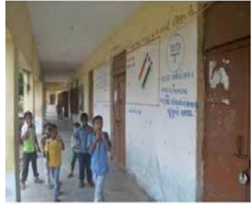
Polling Station Front View
