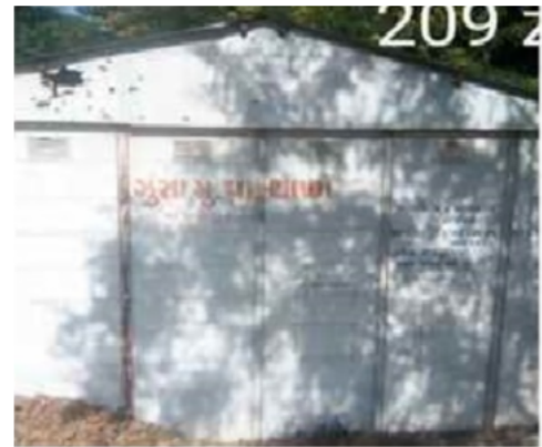
Polling Station Front View
