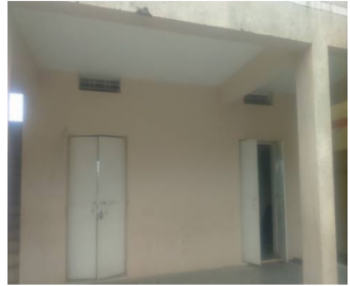
Polling Station Front View
