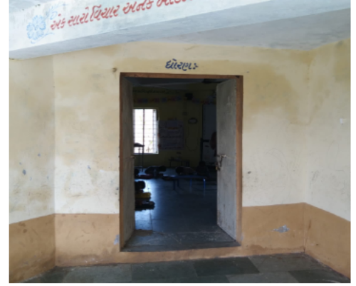
Polling Station Front View
