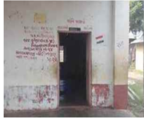
Polling Station Front View
