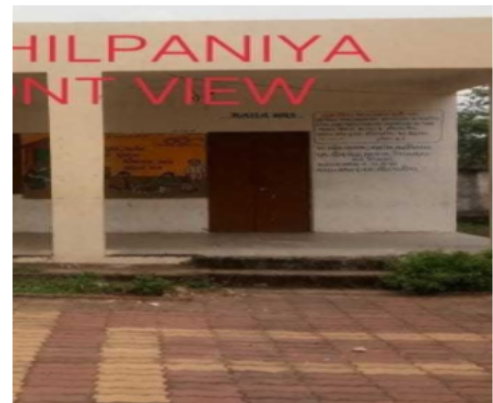
Polling Station Front View
