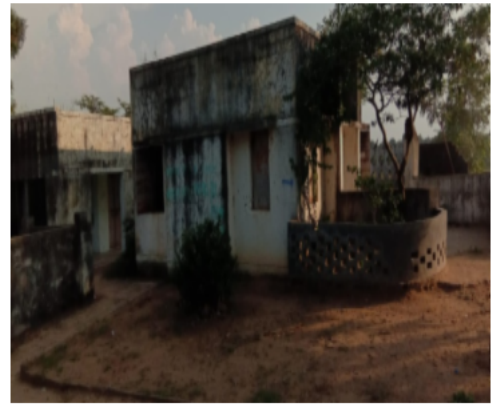
Polling Station Front View
