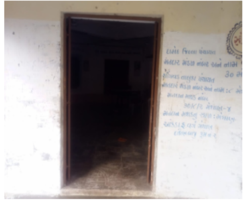
Polling Station Front View
