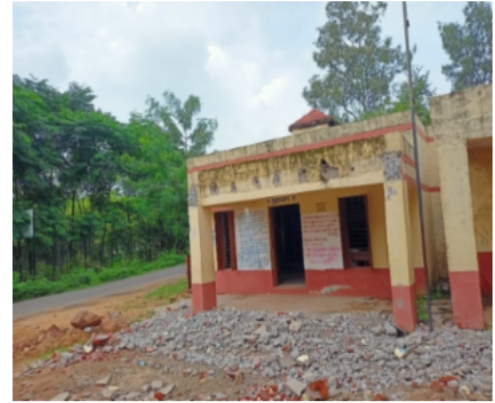
Polling Station Front View
