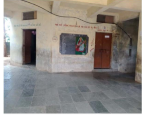
Polling Station Front View
