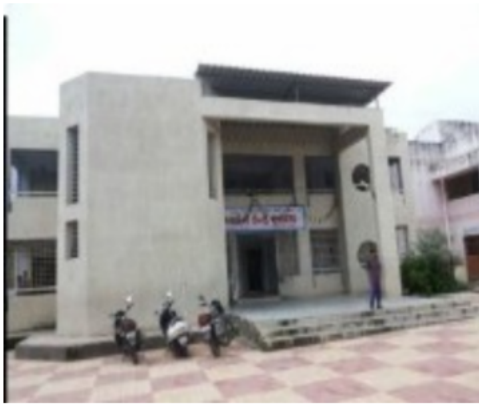
Polling Station Building Front View
