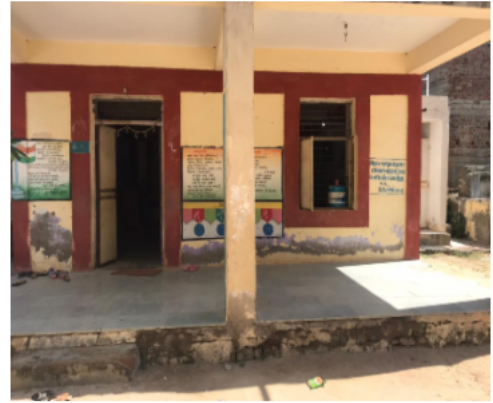
Polling Station Front View
