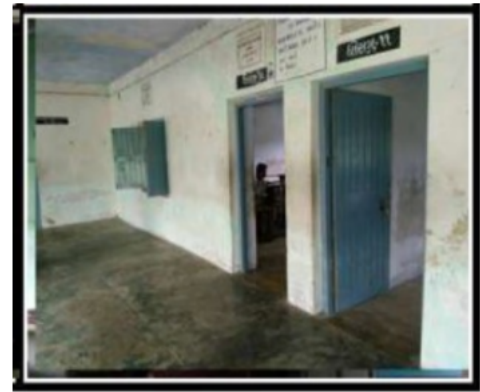
Polling Station Front View
