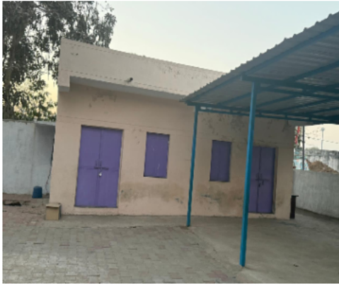
Polling Station Building Front View
