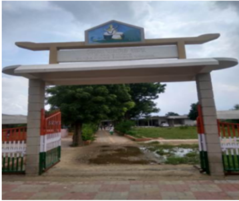
Polling Station Building Front View
