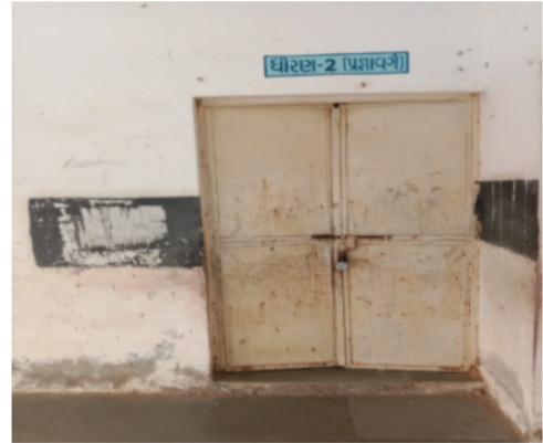
Polling Station Front View
