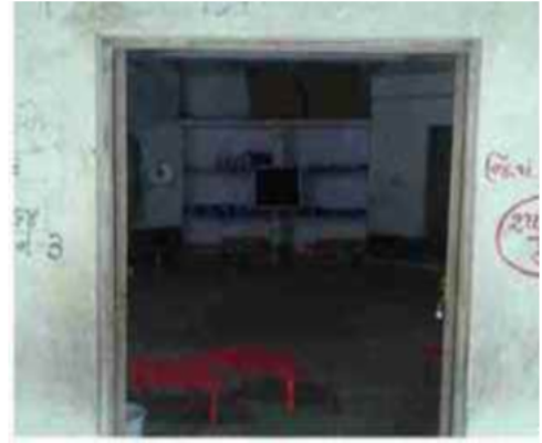
Polling Station Front View
