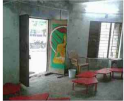
Polling Station Front View
