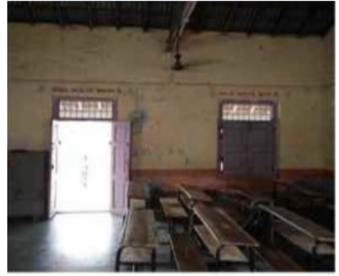
Polling Station Front View
